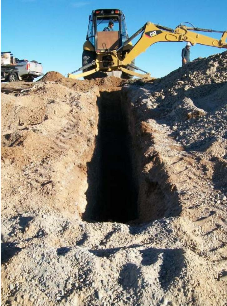
**Exploration at Laguna Salada has been mainly through mechanized trenching due to the unconsolidated nature of the gravel. The uranium-vanadium mineralization at Laguna Salada occurs within a flat layer located within three metres from surface in soft sandy gravel in a semi-desert environment.**
